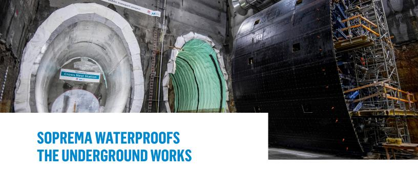
SOPREMA FLAGON PVC tunnelling system was installed in a few of the deepest stations on the city's metro train line, which are expected to host large buildings above the stations: Martin Place, Victoria Cross, Pitt Street, Crows Nest, and Waterloo Station sites.
