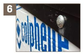
Use a pressure seal termination barre with a bead of SOPRAMASTIC / SOPRAMASTIC ALU to seal the membrane termination
