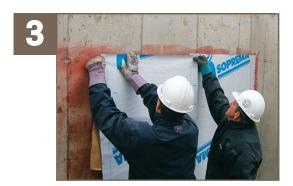
Peel back the top part of the silicone release film. Adhere COLPHENE 3000 to the substrate, making sure the membrane is well aligned.
