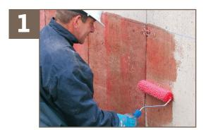
Prime the substrate with ELASTOCOL STICK or ELASTOCOL STICK H<sub>2</sub>O.
