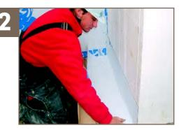
Install a reinforcement strip membrane centered on the corner of all interior and exterior foundation angles.
