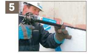
Use SOPRAMASTIC / SOPRAMASTIC ALU to seal details and critical areas. The use of a protection or drainage board is recommended before backfilling to ensure the integrity of the waterproofing membrane.
