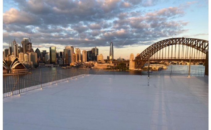
Kirribilli, NSW Synthetic Waterproofing (PVC)
