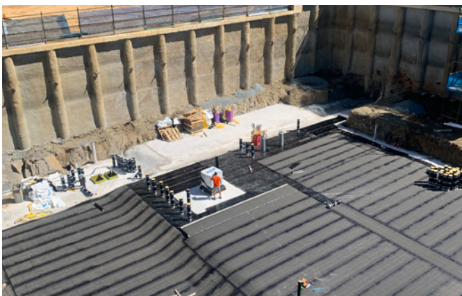
Canberra, ACT Foundations - Pre-applied Blindsided Waterproofing
